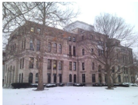
Courthouse with domes removed
