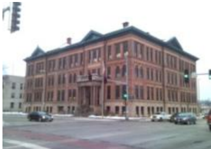
County office building
